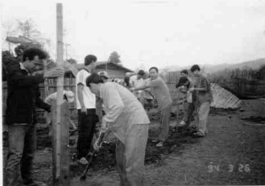
Preparation the land for Building costruction of new CLC in 1994
