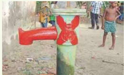
Marking arsenic-contaminated tube wells with paint / ©BRAC
